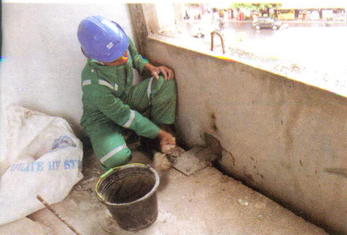
Application for precast gap
